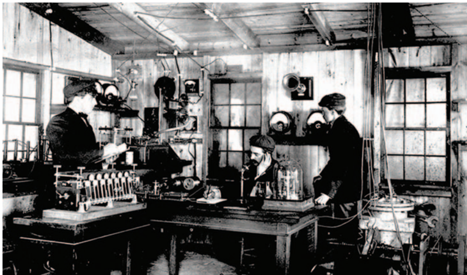
Brant Rock shack in 1906. Adam Stein is on the left of the photo. The RF alternator is lower right, in front of the compressed air tuning capacitor. The receiver is on the left, the loudspeaker on the wall, and the high current telephone relay under the glass dome on the table.
